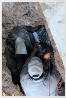
Some sections of the pavement slabs were repaired on Circuito Julio Berdegué Aznar, by homes No. 70, 71, 72, 73, and 80, which included demolition, compacted fill and pouring, as well as new potable water pipes.
